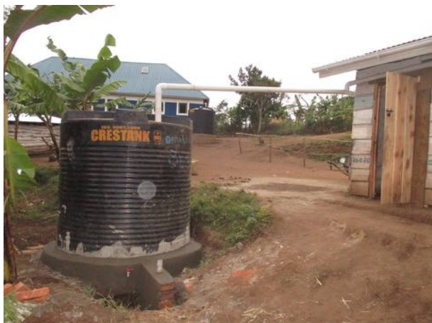
Water tank from old school site installed with guttering on the wooden kindergarten building (June 2017)
